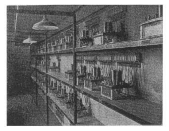
Relay-terminal case on first floor of tower
