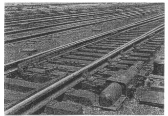
Electro-pneumatic switch movement with CP valve
